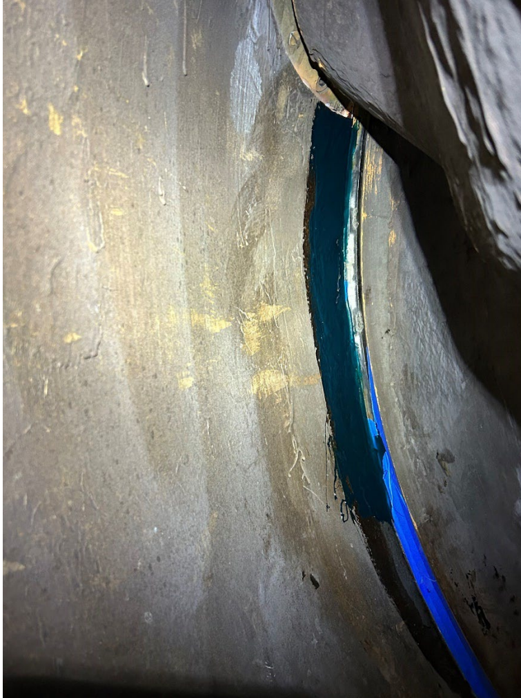
Figure 7.—PE1 is shown applied between the 8 o'clock and 9 o'clock positions.
