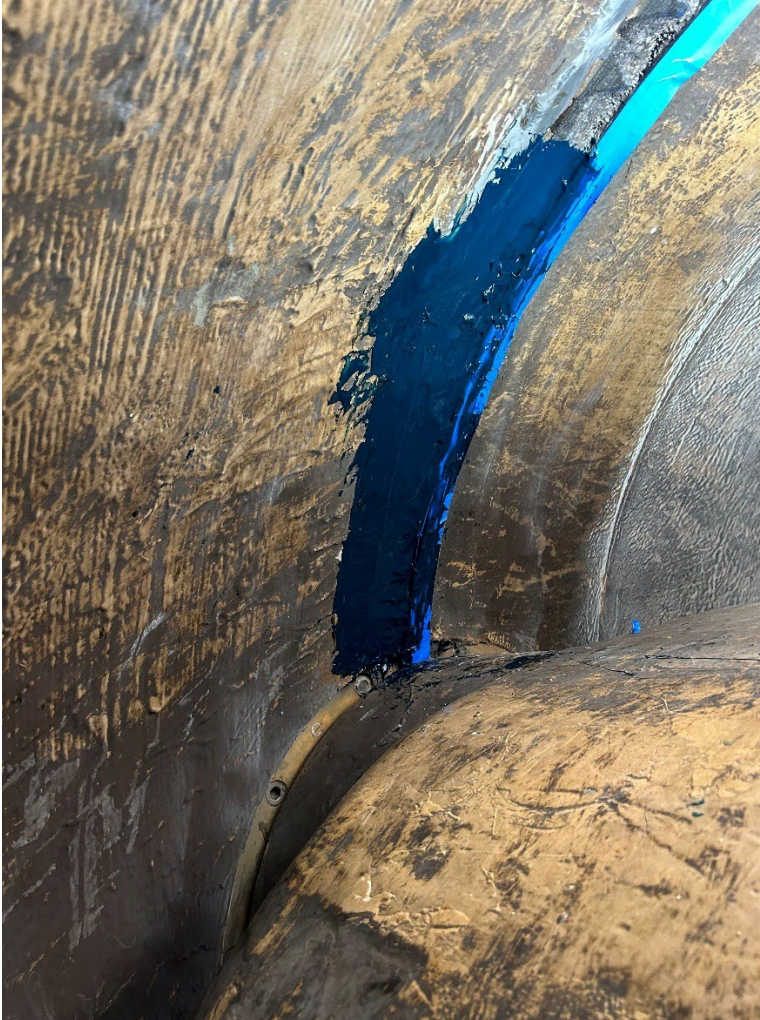
Figure 6.—PE1 is shown applied between the 9 o'clock and 11 o'clock positions.
