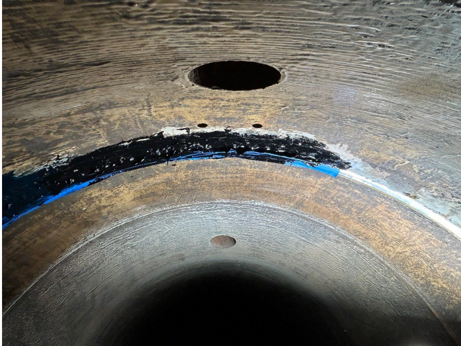
Figure 8.—PE2 is shown applied between the 11 o'clock and 1 o'clock positions.
