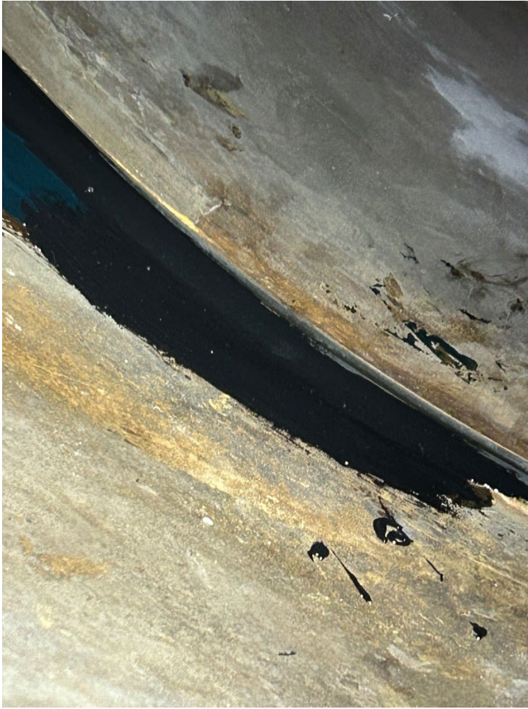
Figure 10.—PE2 is shown applied between the 7 o'clock and 8 o'clock positions.
